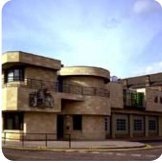
Tollcross Fire Station, Edinburgh
